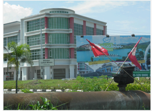
Lahat Mines has now been converted into a resort, commercial and housing area.
