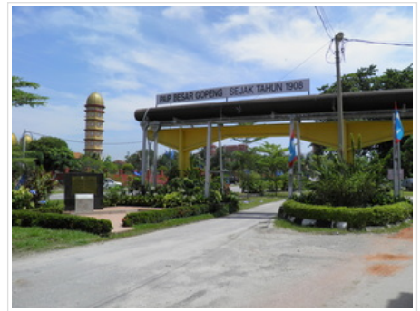
A section of mining pipeline dating from 1908 has been preserved in Gopeng
